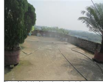
Photo of the inside of the main production hall Edge railing found at roof top.JPG
