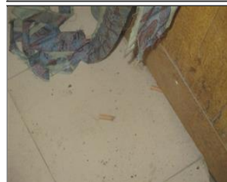
Photo of non-conformity Leftover cigarettes buds found in roof top rest room.JPG
