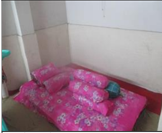
Photo of non-conformity No separte breast feeding facility found at child care room.JPG
